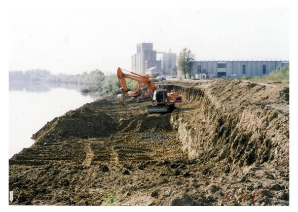
Construction of vertical quay No. 3 in lenght of 120 m with handling and logistics area with total surface of 3.910 m<sup>2</sup>, finished in 2011.
