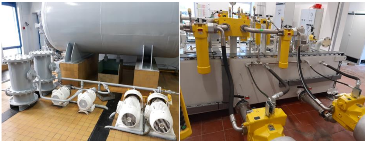
Photo 2: Iron Gate I navigation lock electro-hydraulic features after the performed upgrade
