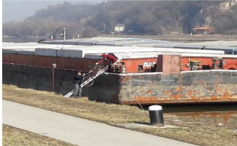
Previous Upgrade in Linz
