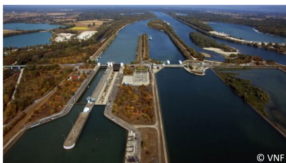
Doubling of locks as backup to avoid disruptions in case of maintenance, incidents and accidents
