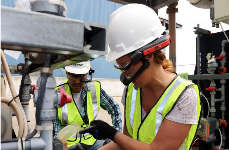
Figure 4: head mounted tablet in use for purpose of remote maintenance
